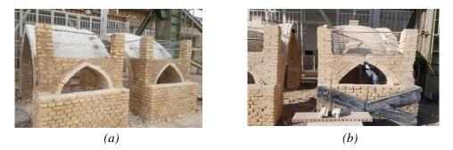
Figure 3. The stages of construction structure: a) Structure view of arch and rib cover; b) Structural view after reinforcement.
