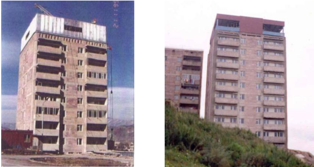
Figure 6. Seismic Upgraded Buildings using AIUF.
