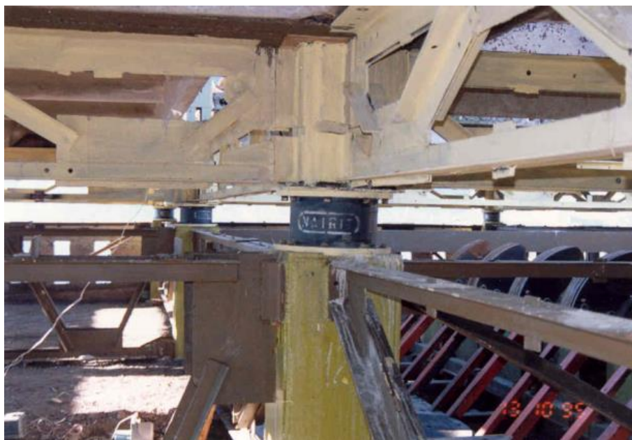
Figure 7. AIUF Implementation Technique on Roof Floor of 111 Series building.
